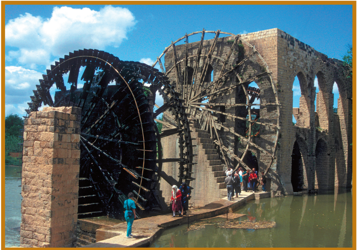
These norias or waterwheels, which raise water from the Orontes River, are in Hama, Syria
